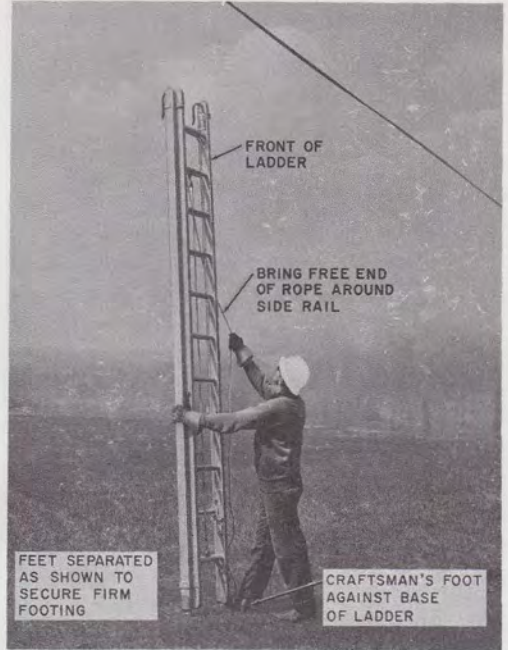
Fig. 13—Preparing to Extend Top Section
