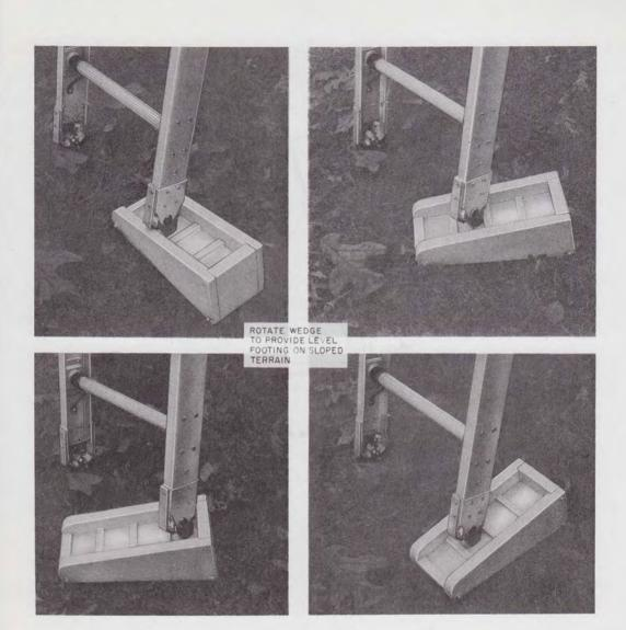
Fig. 11—B Ladder Leveling Wedge in Use
