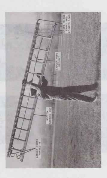
Fig. 6—One-Person Method of Carrying an Extension Ladder
