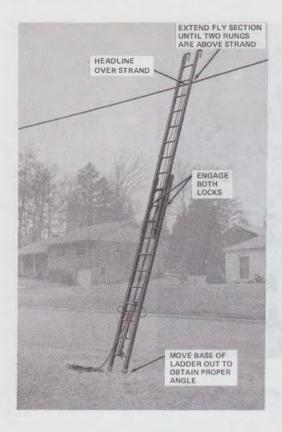
Fig. 21—Ladder in Working Position
