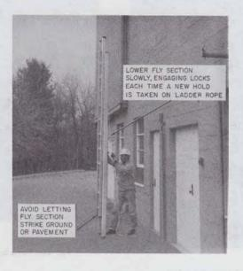
Fig. 26—Fly Section Lowered
