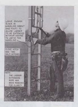
Fig. 20-Method of Securing Handline
