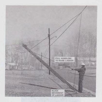
Fig. 18—Ladder Partially Raised
