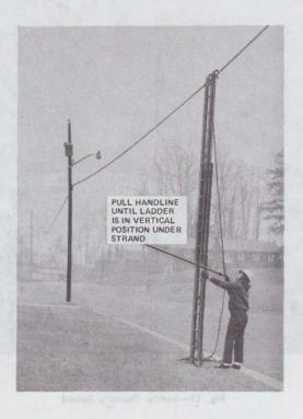
Fig. 19—Ladder in Vertical Position
