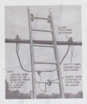
Fig. 45—E Ladder Support in Position on Strand
