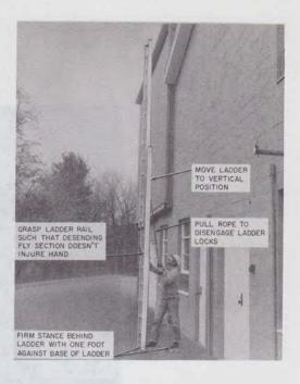
Fig. 25—Preparing to Lower Fly Section
