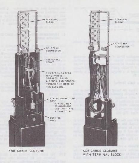
Fig. 18— Service Wire Installed—K Type Cable Closure (Protected)
