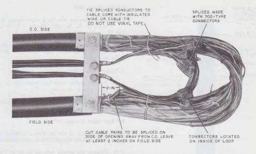
Fig. 6-Wire Work Completed-14-Type Closure
