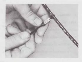
Fig. 2—▶Placing Tie and Marker¶
