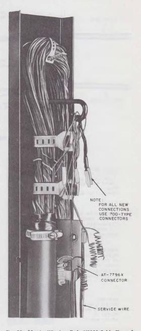
Fig. 22—▶Service Wire Installed—UP200 Cable Closure◆
