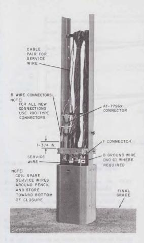
Fig. 20—♦Service Wire Installed—LD Type Cable Closure♦
