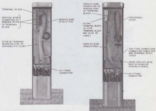
Fig. 10—\$Service Wires Terminated in PC6/48 Cable Closure—Fixed Count Mode\$
