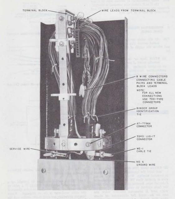
Fig. 16—♦Service Wire Installed—J Cable Closure (Protected)♦
