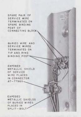
Fig. 24—♦Service Wire Terminated—D or E Buried Wire Terminal♦
