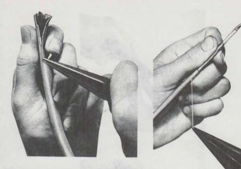
Fig. 5—♦Stripping D Inside Wiring Cable or G and H Station Wire (With Jacket-Slitting Cord)♦
