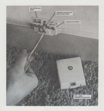
Fig. 12—No. 723 Terminal Base With W.E. 625C Connecting Block
