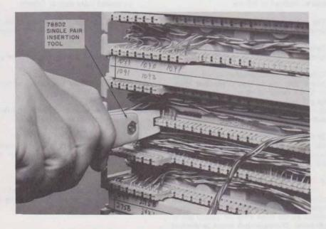
Fig. 26—Seating Conductors With Single-Pair Insertion Tool
