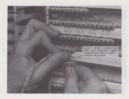
Fig. 21—Inserting Cross-Connect Wire
