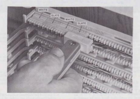
Fig. 19—Seating Connecting Block on Index Strip
