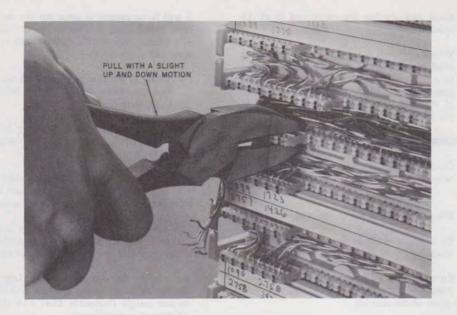
Fig. 25—Removing Connecting Block
