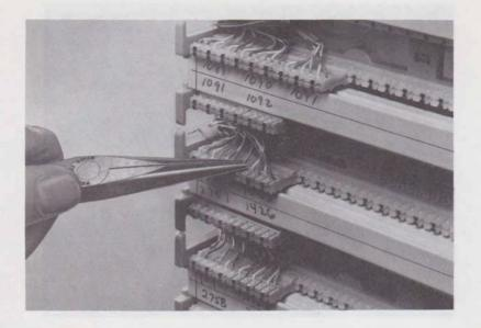
Fig. 23—Removing Cross-Connect Wire
