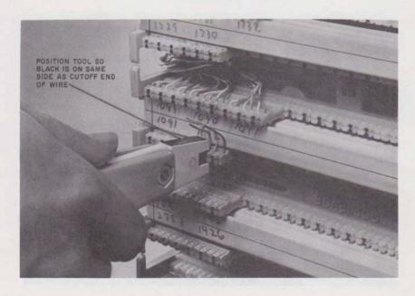
Fig. 22—Terminating Cross-Connect Wire
