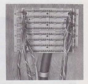
Fig. 13—200-Pair Cable in Cable Slots
