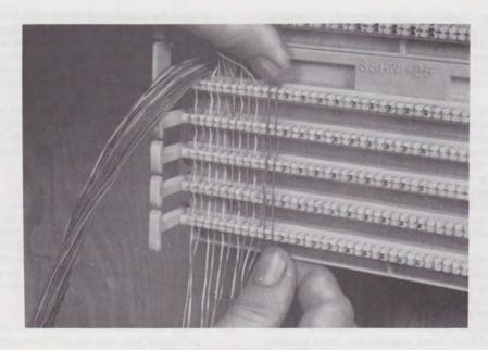
Fig. 16-Multiple Connections in Red Field
