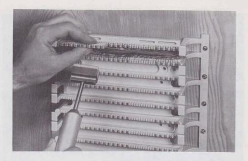
Fig. 18—Connecting Block Placed on Index Strip
