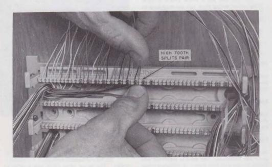
Fig. 14—Placing Conductors in Index Strip
