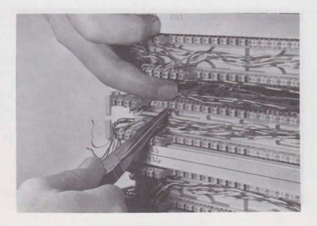
Fig. 24—Reterminating Cross-Connect Wire
