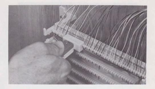
Fig. 15—Seating Conductors in Index Strip
