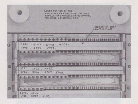
Fig. 20—Marked Designation Strips on Wiring Block
