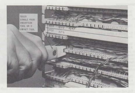
Fig. 27—Seating Conductors With Single-Pair Insertion Tool
