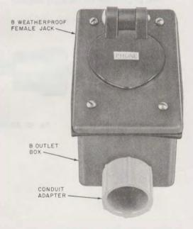
Fig. 48—B Weatherproof Female Jack on B Outlet Box
