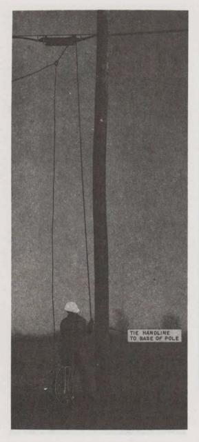
Fig. 6—Drop Wire Raised to Approximate Height
