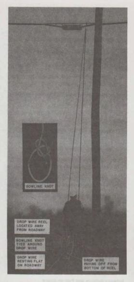
Fig. 4—Bowline Knot Placed Around Drop Wire
