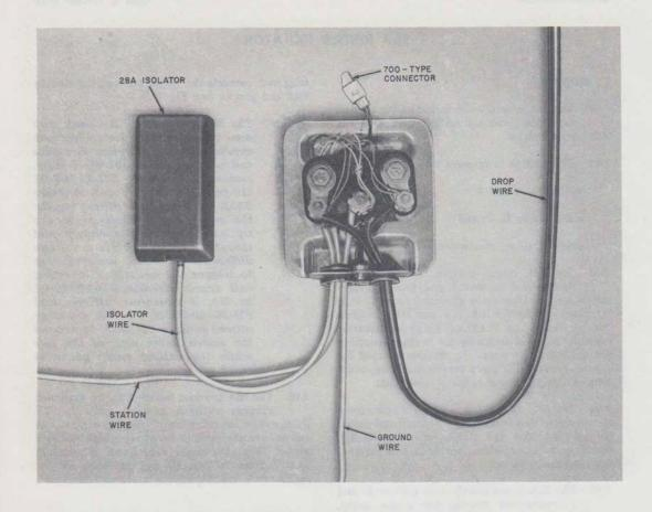
Fig. 1—28A Ringer Isolator, Typical Installation
