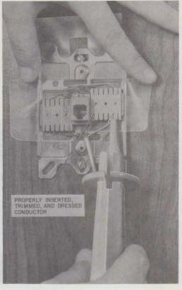
Fig. 17—Connecting Wire With Lead Insertion Tool
