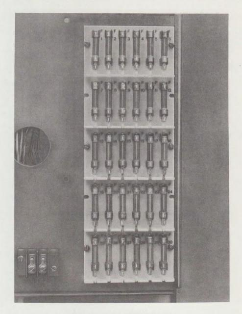
Fig. 7—Fuse Panel on 2-Type Power Panel
