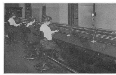
Figure 19. Typical installation of Cordless B positions in a machine sw
