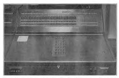
Figure 18. Incoming trunk position ("cordless'B") in a machine switching office.
