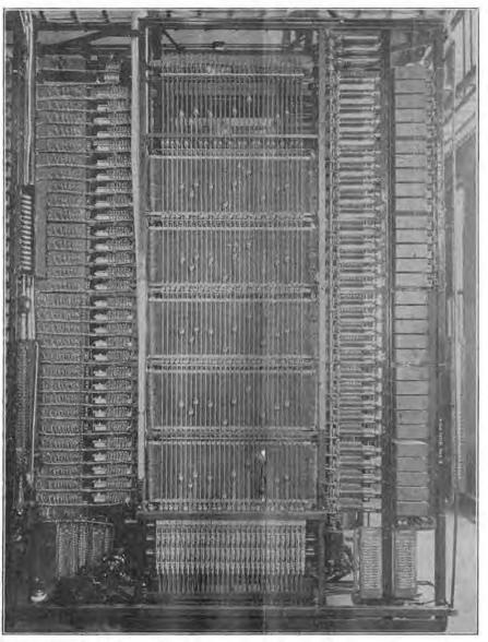
Figure 8. Typical selector frame showing general arrangement of district, office, incoming and final frames.
