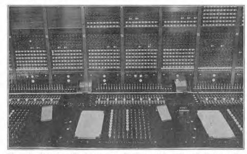
Figure 16. Manual position in automatic office arranged for semi-mechanical operation.
