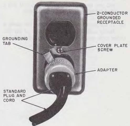
Fig. 10—Grounded 2-Conductor Receptacle
