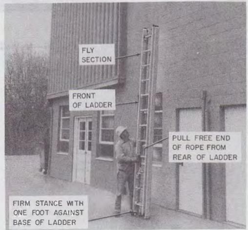
Fig. 23—Preparing to Extend Fly Section
