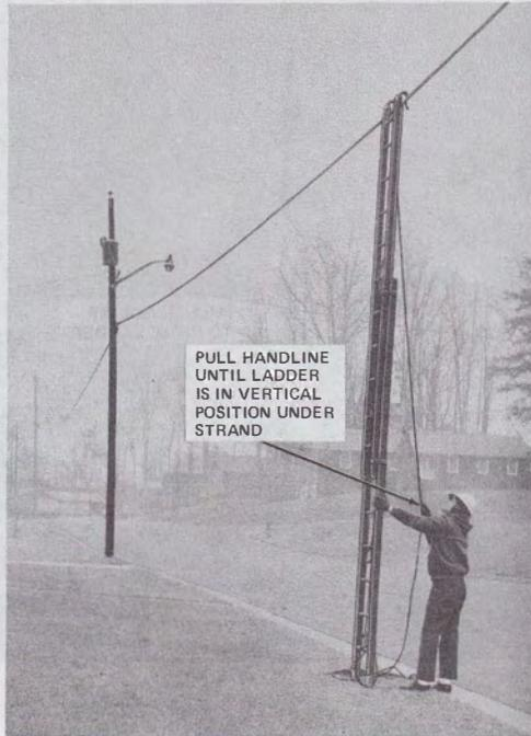
Fig. 19—Ladder in Vertical Position
