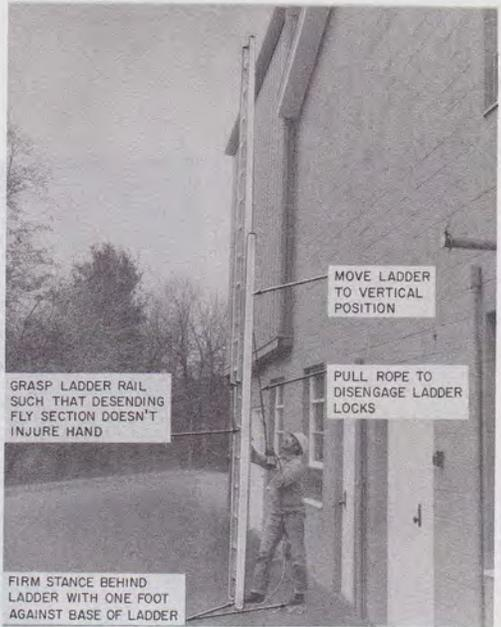
Fig. 25—Preparing to Lower Fly Section
