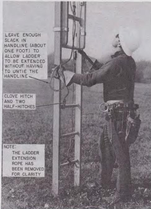
**Fig. 20—Method of Securing Handline**
