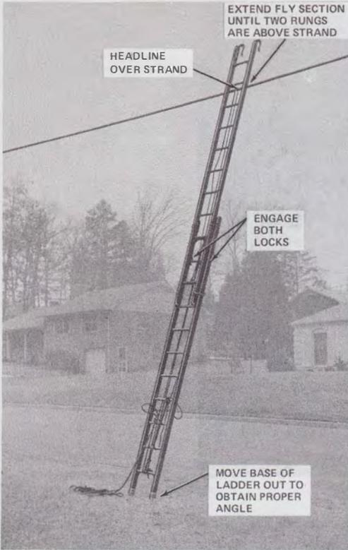
Fig. 21—Ladder in Working Position
