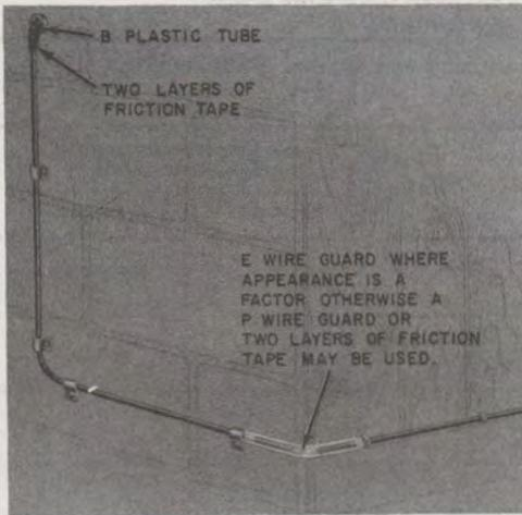
Fig. 2—Use of Tape or E Wire Guard
