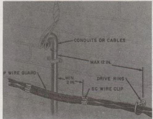
Fig. 12—Wires Crossing Cables, Conduits, Signal, or Ground Wires on Masonry or Brick Surfaces
