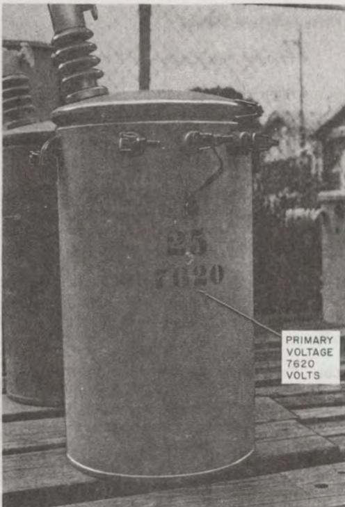
Fig. 9—Voltage Marking on Transformer
