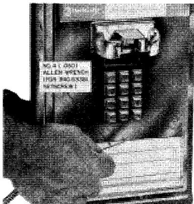
Fig. 21—Securing Instruction Card (Typical)
