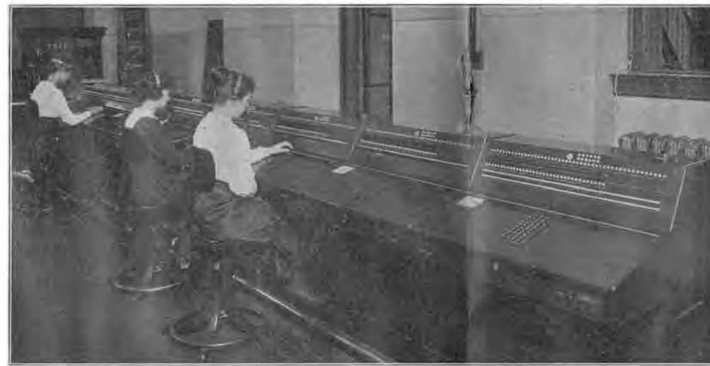
Figure 19. Typical installation of Cordless B positions in a machine switching office.
