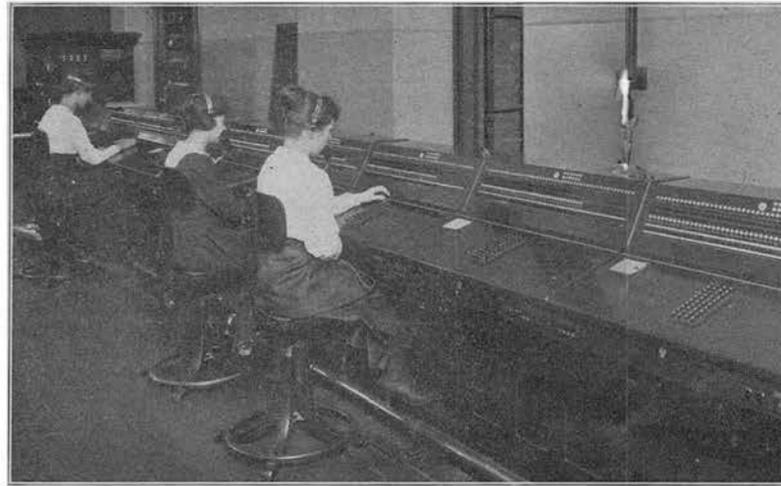
Figure 19. Typical installation of Cordless B positions in a machine switching office.
