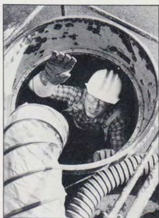
George Dembzyński, Turnersville installation and maintenance
