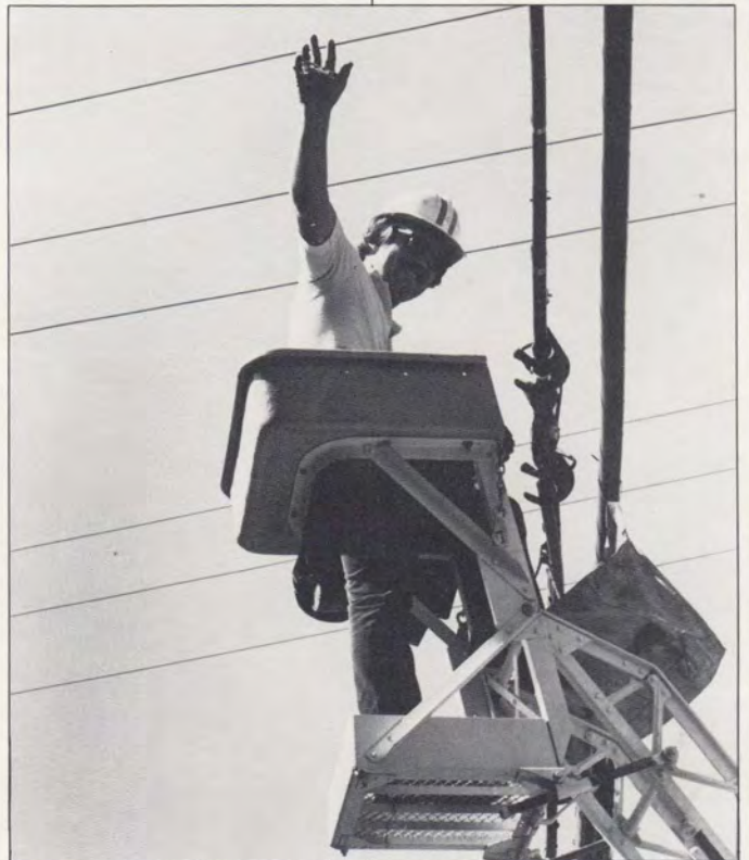
Paul May, Burley installation and maintenance
