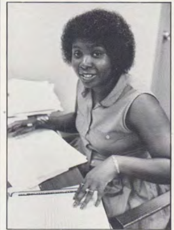
Priscilla Thomas, Newark toll equipment center
