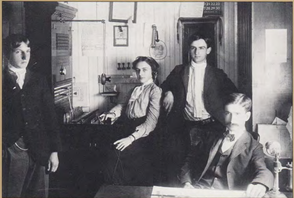
One of the early switchboards—Gerard's Drug Store, Rockaway, N.J., 1903.
