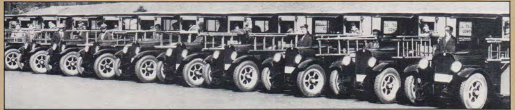
Installation trucks, circa 1930.
