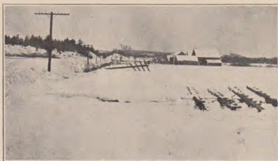
EIGHT MILES OF WIRE DOWN AFTER THE STORM
