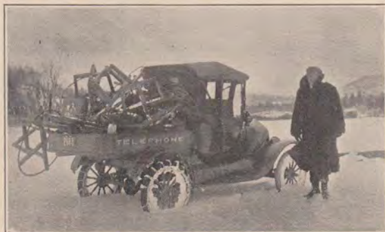
CHISHOLM AND "HENRY" READY TO RUN PERMANENT WIRE ON TOLL SECTION 143
