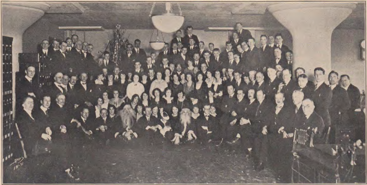
THE PLANT FOLKS AT STATE STREET HAD A REGULAR TIME, DECEMBER 24
