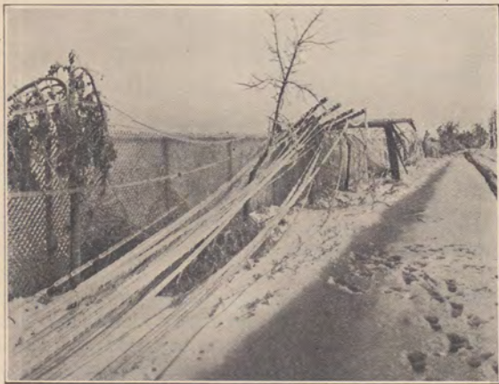
JUST ONE OF MANY This pole carried our Boston to Worcester circuits. West of Framingham Junction, twelve poles like this were blown down.
