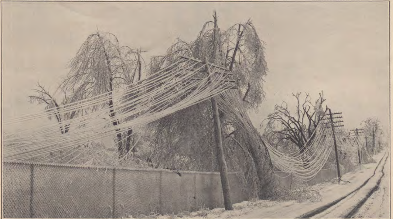
WHAT THE WORST STORM IN TELEPHONE HISTORY DID NEAR FRAMINGHAM Note the twisted crossarms and sagging wires on which rested ice-covered tree limbs.
