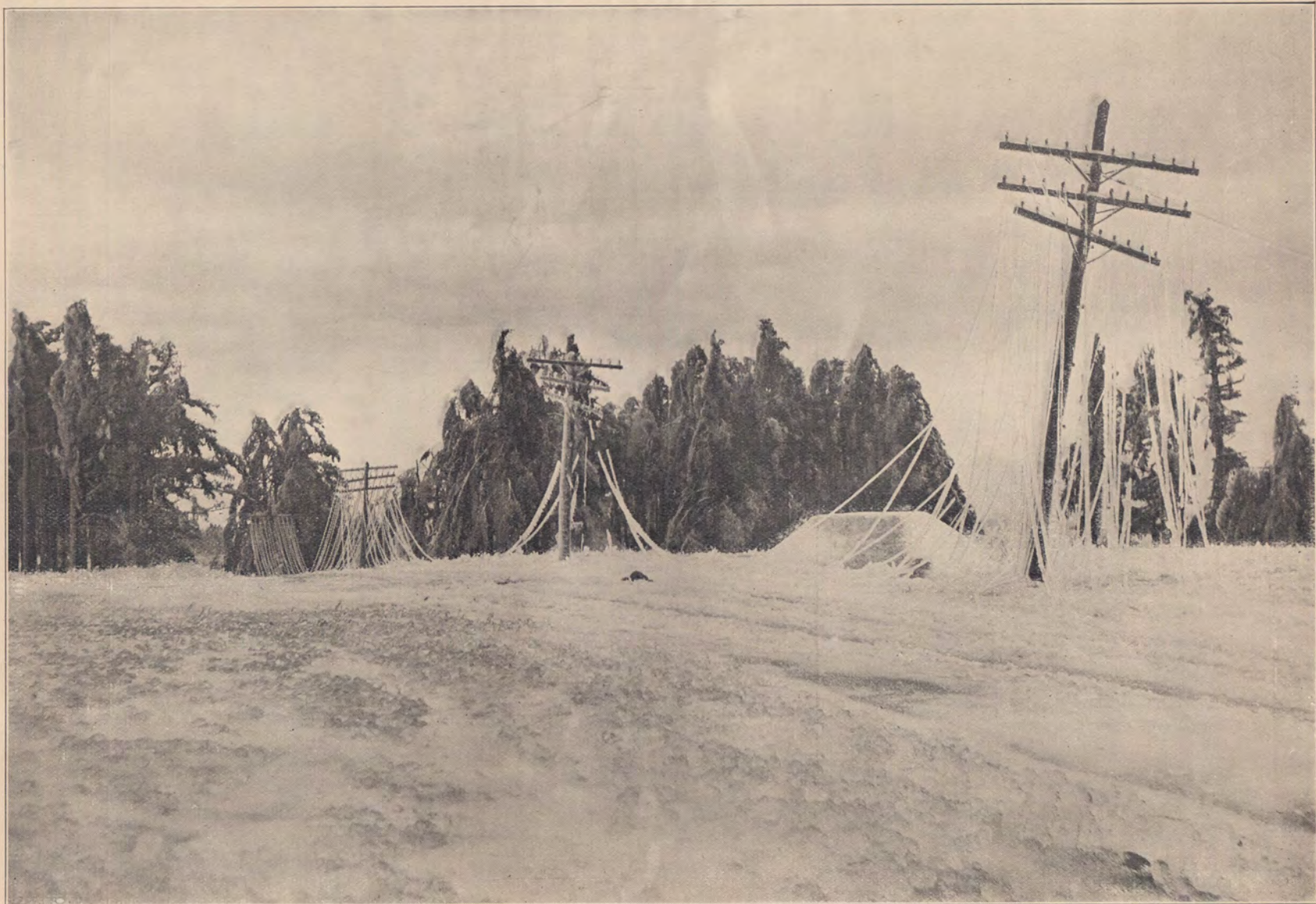
DOWN AND OUT, BUT ONLY TEMPORARILY Toll Section 70, near Chester, Mass.
