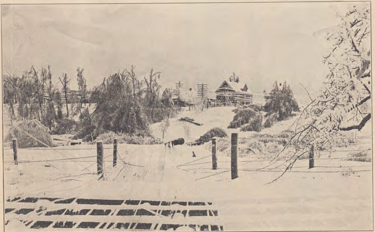
STORM DAMAGE AT WORCESTER
