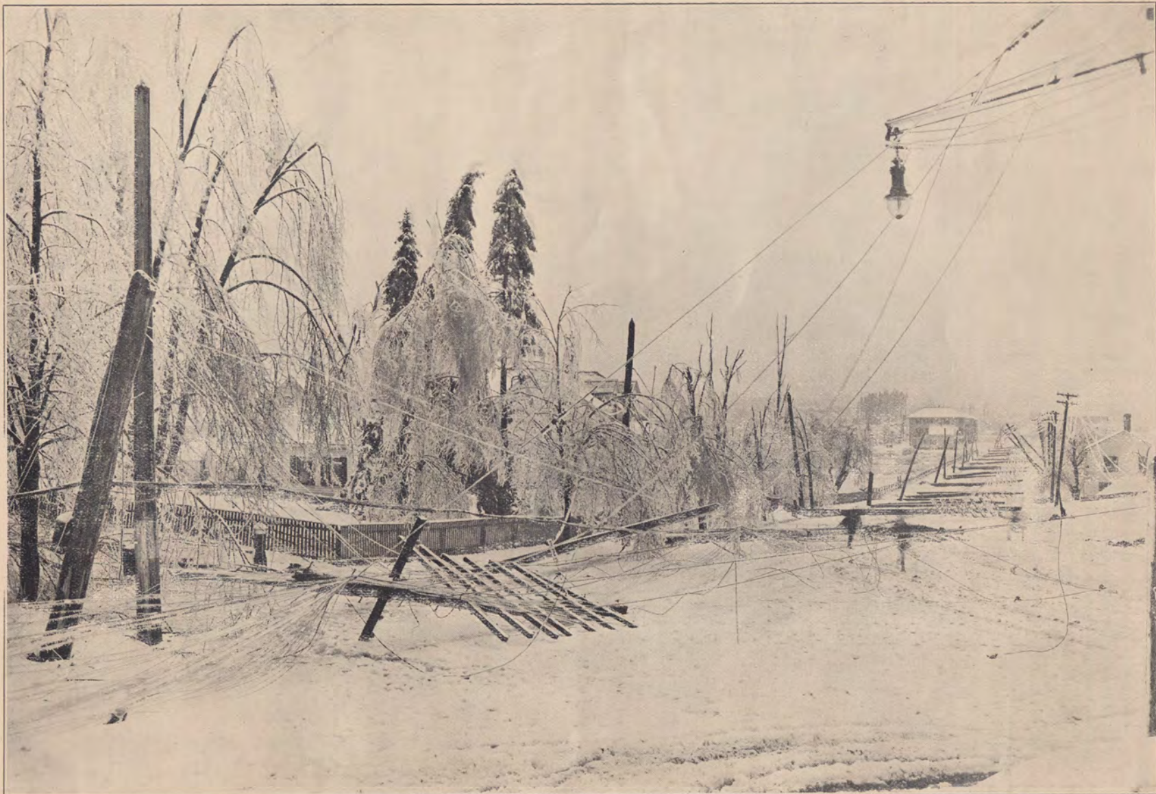
IN SOME PLACES AS FAR AS THE EYE COULD SEE, POLES WERE DOWN Worcester suffered severely from the storm, as witness this picture taken of Stafford Street, near Ludlow Street, Worcester
