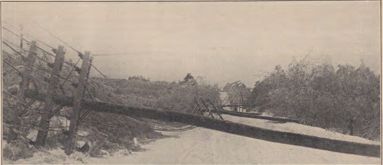
A detour was necessary on Green Street, Woburn, because fallen telephone poles blocked the street.
