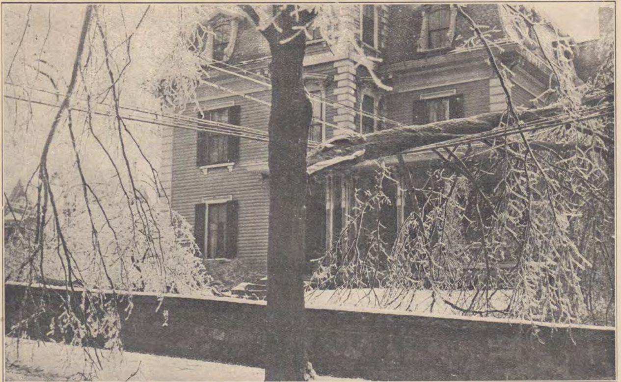
FALLING TREE LIMBS CAUSED GREAT DAMAGE The limb shown in the picture destroyed many local lines in Stoneham, in addition to our Stoneham-Woburn Cable.
