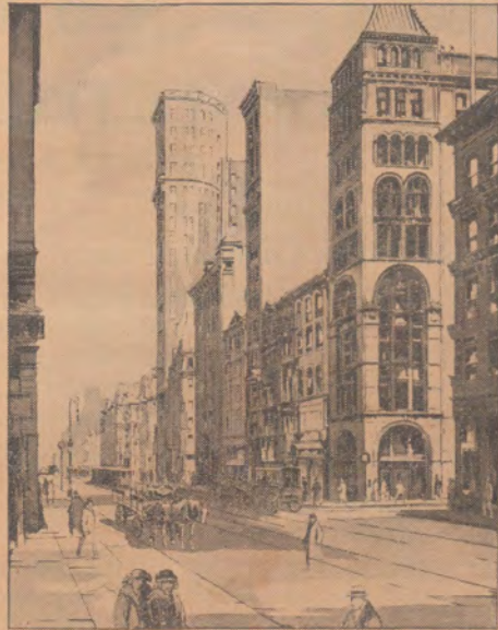
The same scene after the overhead wires were replaced by underground cables
