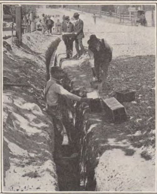
C. A. MATTESON GIVES RESERVOIR AVENUE CONDUIT JOB THE "ONCE OVER"
