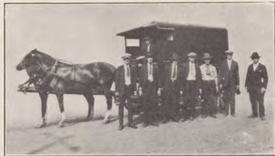
THE SUBSTATION INSTALLATION GANG
