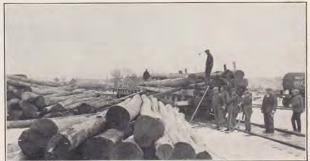
GETTING READY FOR A BUSY CONSTRUCTION SEASON AT BROCKTON
