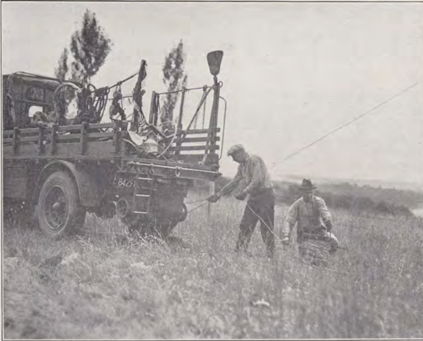
PULLING IN ANOTHER LINK OF COMMUNICATION
