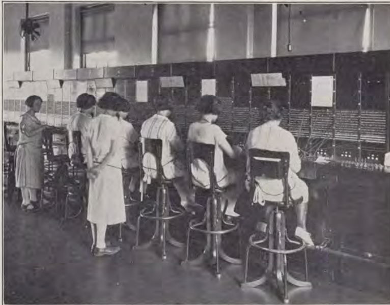
WORKING ON THE NUMBER 11 "A" BOARD AT WELLESLEY
