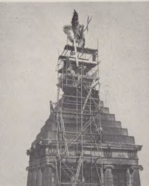
The Spirit of Communication atop the A.T.&T. building in New York had visitors recently who gave the 16-ton statue its periodic inspection. The 27-year-old symbol had its gold leaf coating touched up and stands forth in gleaming splendor.
