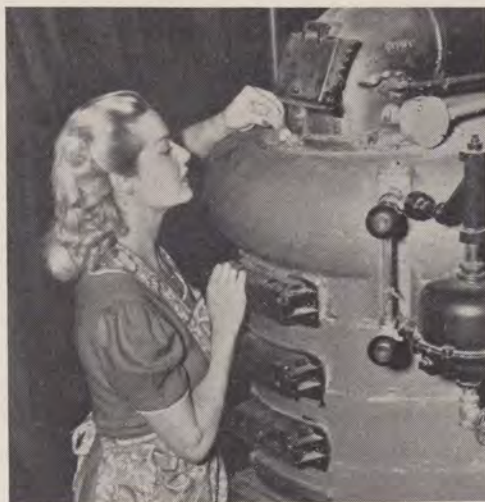
Air leaks reduce heating efficiency and waste fuel. Here the flame of a lighted candle is used to find them. When the flame is drawn into the furnace, the lady has found a leak. It's easily sealed with furnace or asbestos cement.
