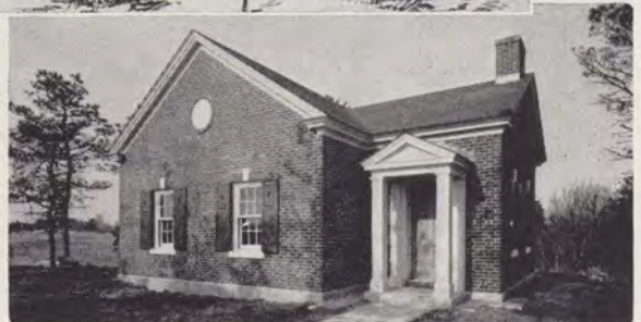
This community dial building in Manomet will house 355A type dial equipment replacing the present common battery type office now in leased quarters.
