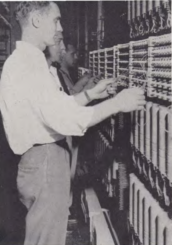
These telephone men, left, are poised, ready to pull the shims to put the new equipment into operation the moment the signal is given at the climax of the conversion.
