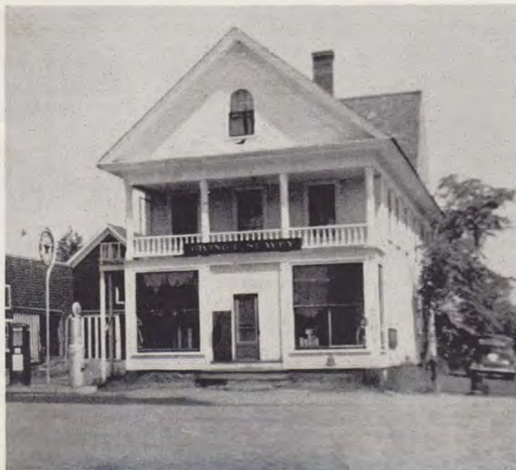
General Store and Telephone Exchange
