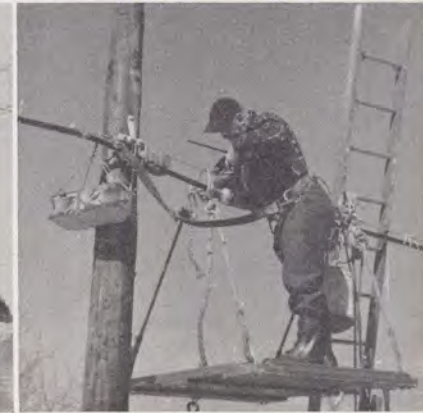
Completing a splice on new light weight alpeth cable at Argyle on the Bangor-Presque Isle route.
