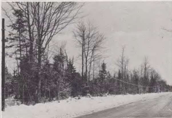
Averaging ten poles per mile, this long span construction on the Bangor-Presque Isle cable route is in Haynesville Woods.
