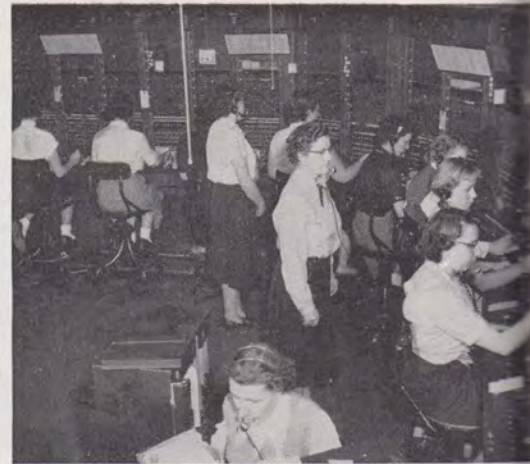
Part of the 14-position manual switchboard of the Brunswick Central Office.
