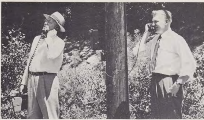
R. B. Meader, Radio Transmission Engineer, was in constant communication by radiotelephone with the helicopter and the hilltop, over a mile away, while D. E. Anderson relayed messages by wire circuit to roof of our Franklin St. Building.
