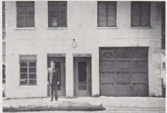
NAVY LT. HENRY J. HOGAN, JR., formerly R. I. Dist. 1 Traffic Manager, sent us this snap of himself standing in front of the Kodiak, Alaska, Telephone Exchange, which he called, "one of the better buildings in this thriving metropolis."
