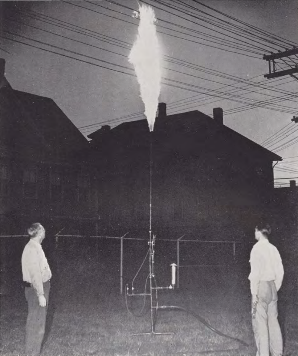
A Christmas tree purge burner lights the early dawn as manufactured gas is burned off to make way for natural gas turned in at 7:00 A.M. on "C" Day.
