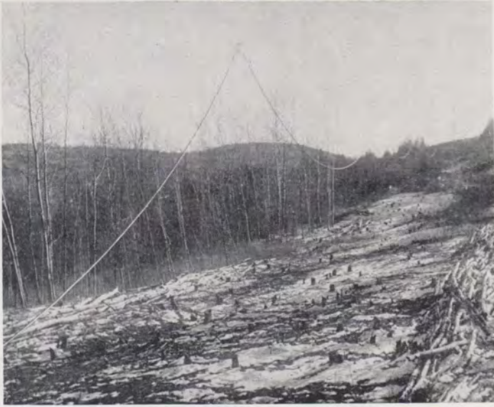
Right: Aerial cable being spliced on the ground thus eliminating necessity of erecting ladders and an aerial platform.
