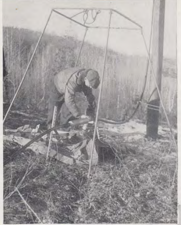
Right: Aerial cable being spliced on the ground thus eliminating necessity of erecting ladders and an aerial platform.
