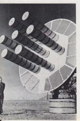
The odd-looking dish with barber poles appended is not some giant telephone cable of the future in cross-section. It's an "apota." Anyway, that's what they call it at Sandia Laboratory in New Mexico, where Western Electric and the Bell Laboratories direct work on military applications of atomic energy for the government. "Apota" is their contraction of "Automatic Positioning of Telemetering Antenna," and undoubtedly the thing is just as complicated as it looks and sounds.
