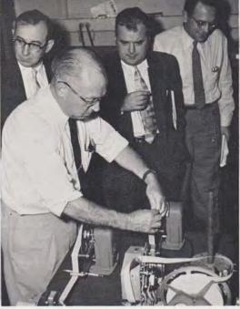
In New York, B. Farrell of the A. P. prepares to feed tape through a reader for transmission to Boston. The second picture taken in Boston shows C. H. Godfroy, Teletypesetter Corporation, removing the tape from the tapewinder to send it to the linecasting machine which puts it into lines of type. Below: a member of the Herald-Traveler staff watches at his linecasting machine as the tape moves from the Teletypesetter attachment on the machine back into the tapewinder to the right.
