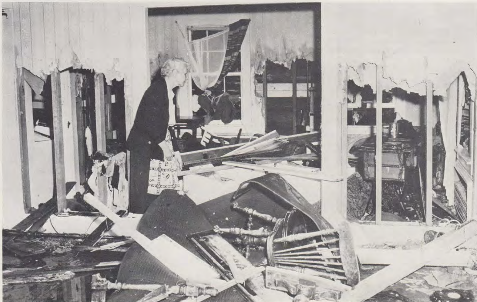
Mrs. Nina Brown, Postmistress of the Swifts Beach Sub-Station, looking over the damage to her home.
