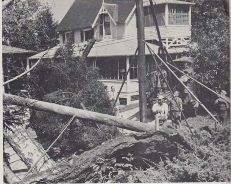
Telephone men work to clear some of the close to 4,000 telephone poles knocked down by Hurricane Carol.
