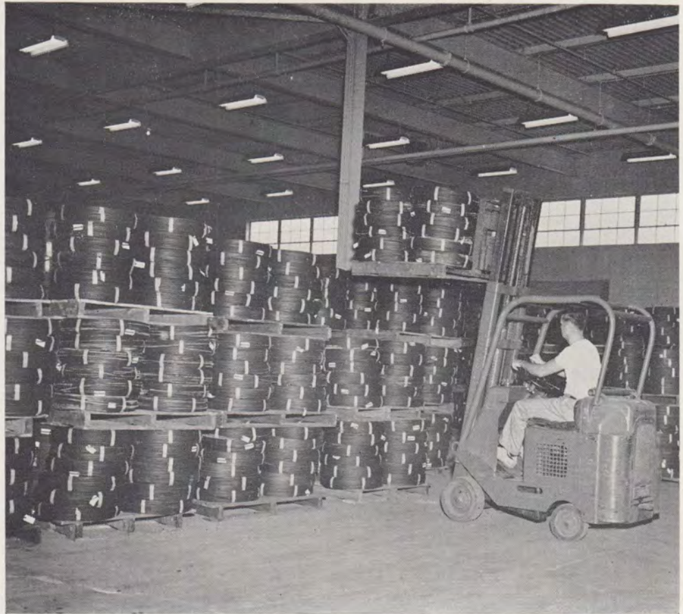
Here's only part of the 14,000,000 feet of drop wire shipped throughout New England from Western's Watertown warehouse in the days that followed the hurricane. This wire is the first link between the subscribers' premises and the rest of the telephone world.
