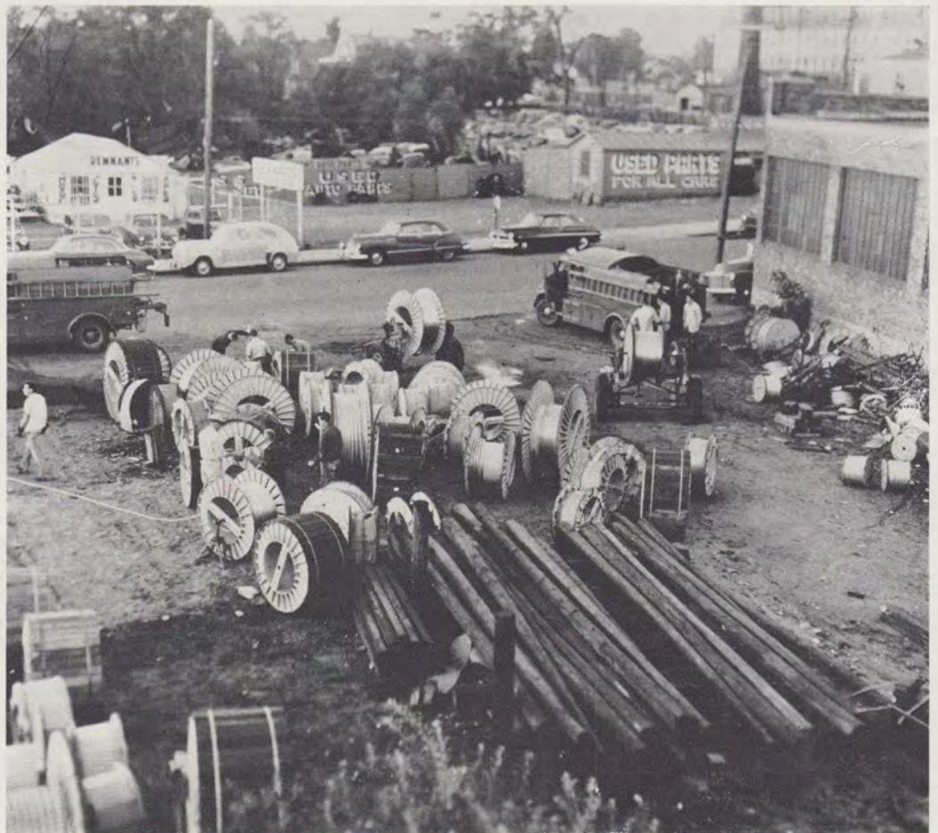
This work operation took place at Framingham as emergency crews picked up materials and supplies at depots established by Western Electric. Emergency equipment of all types flowed into New England from 83 locations in 22 states. The marshalling of manpower and supplies made the telephone restoration job the fastest in telephone history.
