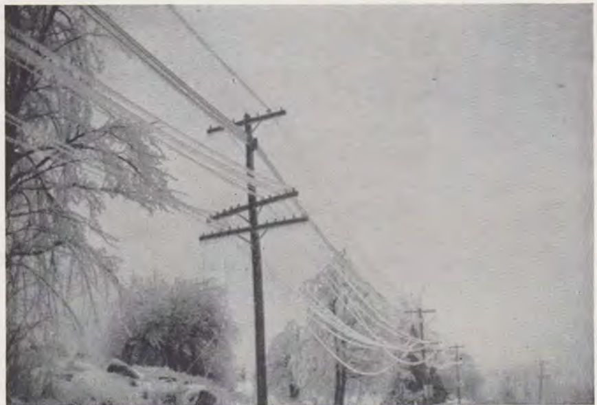
SNOW AND ICE coated these telephone wires along Route 18 in Windsor, Mass. Scenes like this were common sight after the three storms of March 16, 19, and 24 in three-state area. Emergency climbing crews were kept busy restoring power to otherwise isolated homes.
